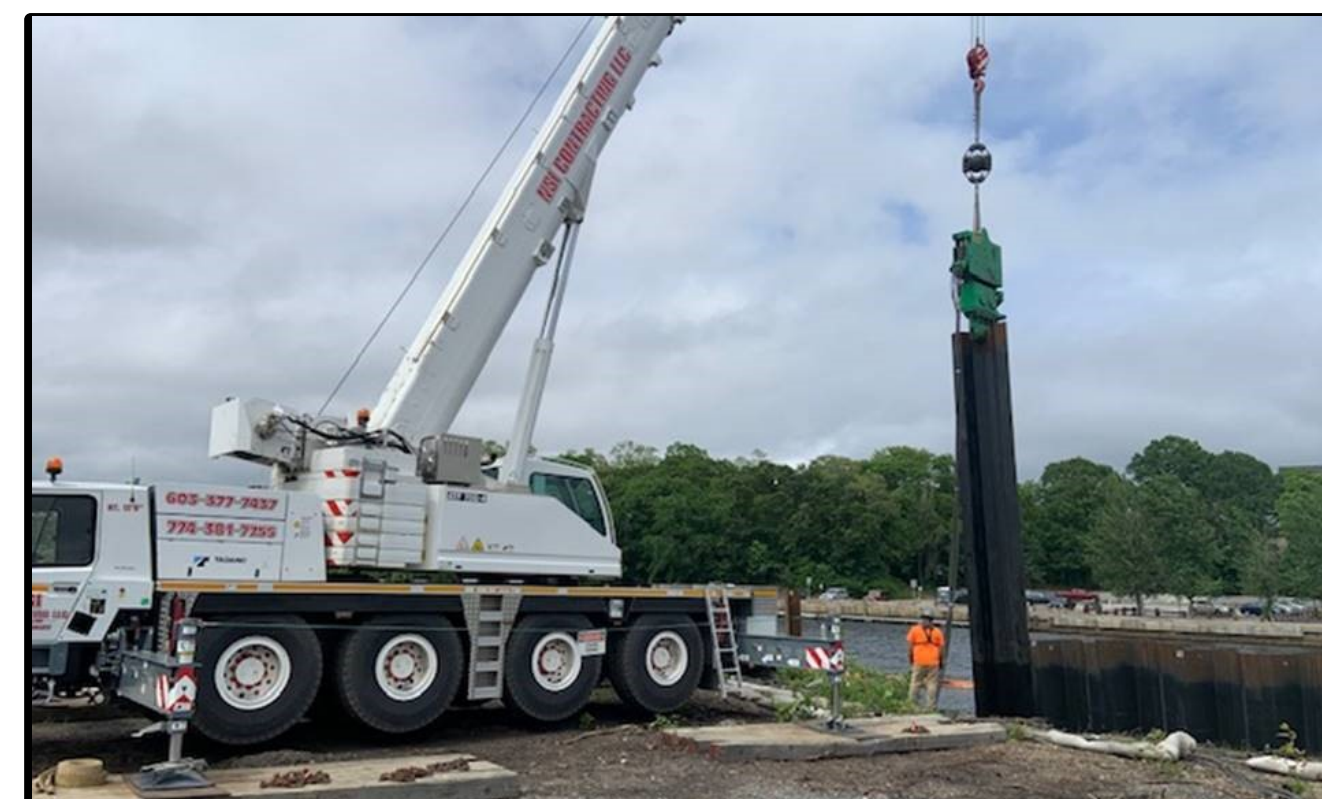
Construction of Barrier Wall - Sheet Pile Installation
