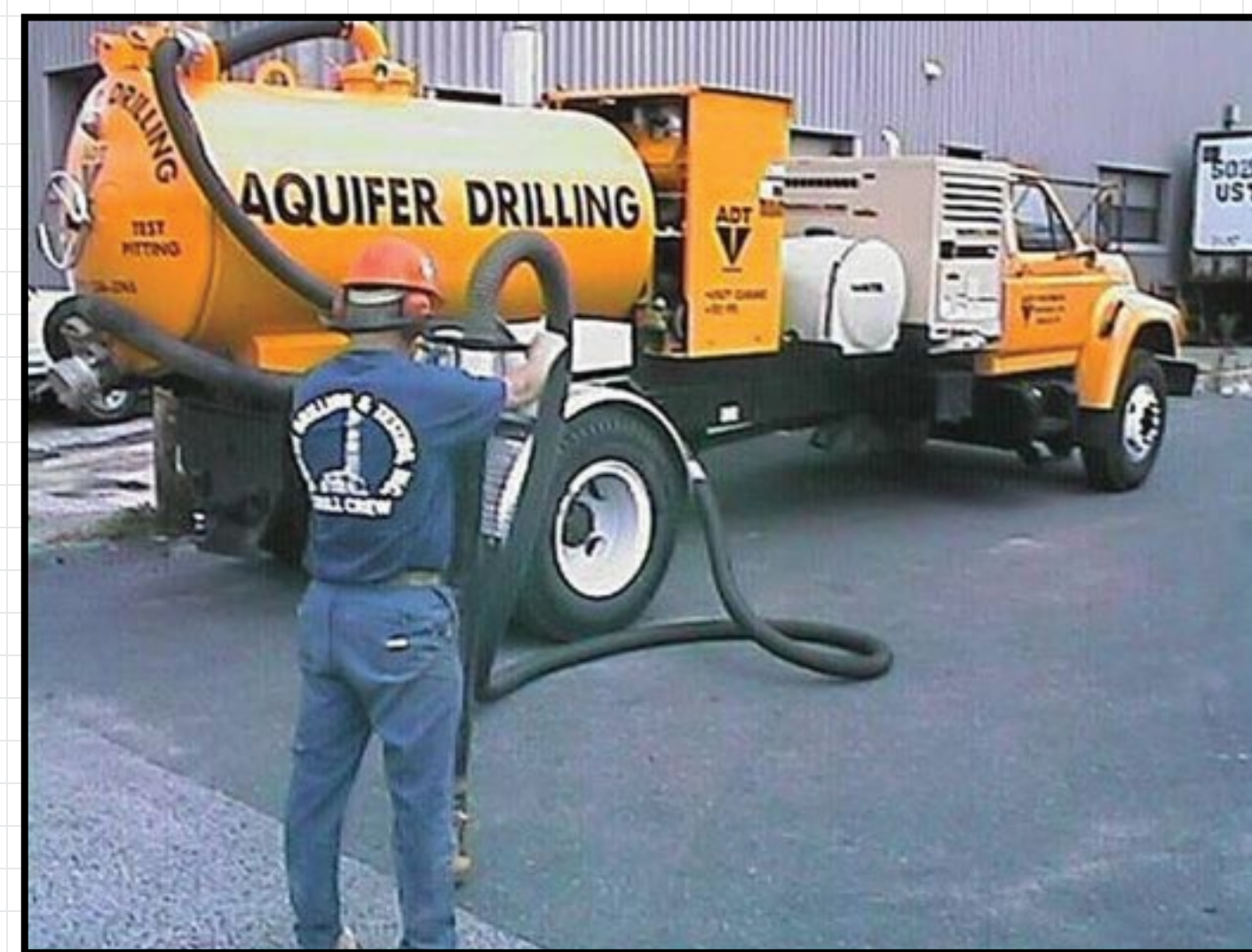
Typical vacuum truck used to remove soil and groundwater
