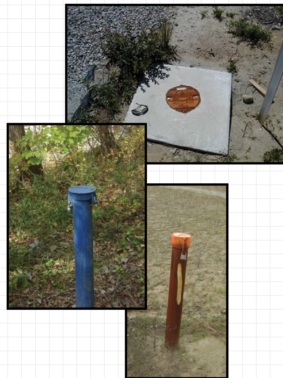
TOP: Typical flush-mounted groundwater monitoring well
