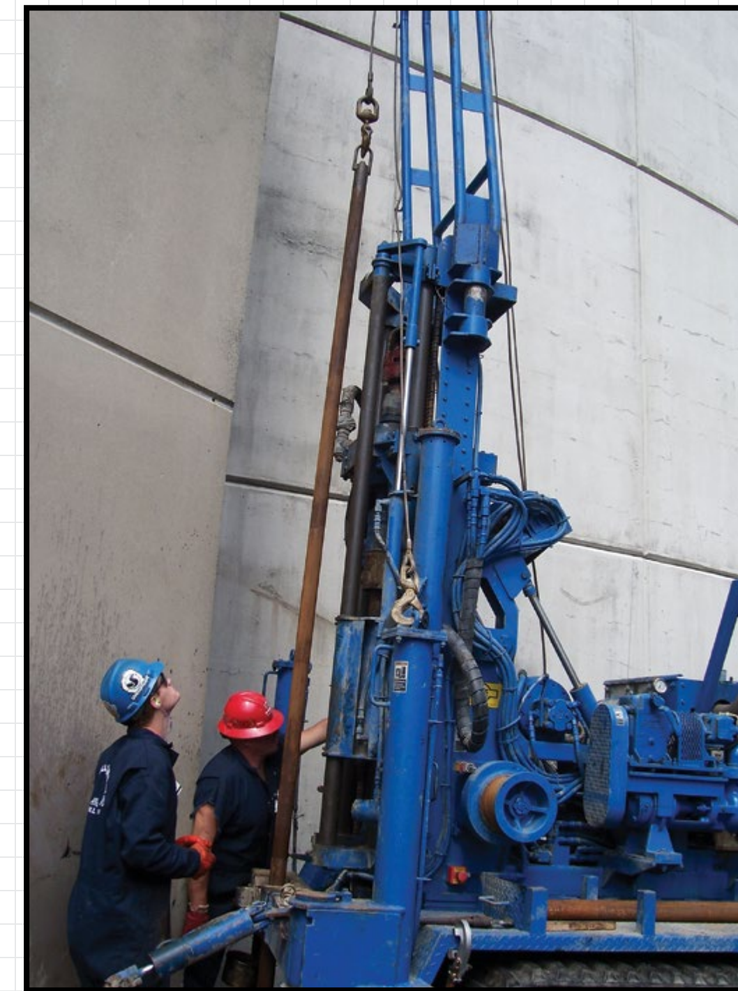
Typical subsurface exploration drilling rods used to collect soil samples
