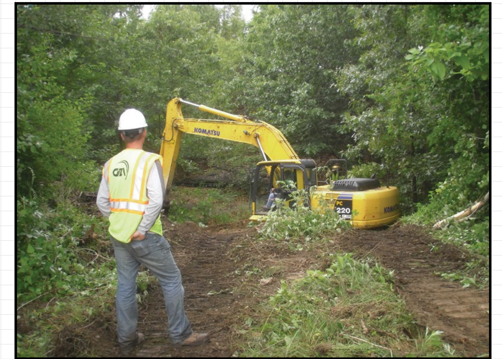
Typical test pitting activities
