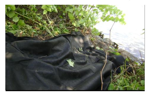
Geotextile placement over area of soil removal. August 23, 2011. 12:46 pm.
