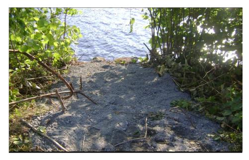
Crushed stone placement over excavated area and geotextile. August 25, 2011. 8:17 am.
